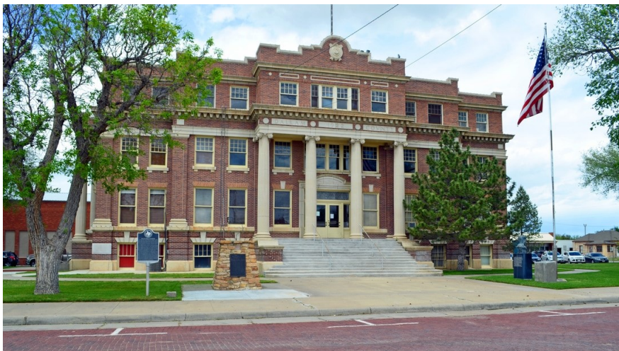
3rd Dallam County Courthouse —1922
